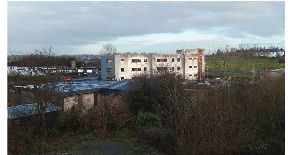
Our intent was to include a photomontage from the edge of St. Mary's Church grounds, as it is a Protected Structure and forms the outer extents of the ACA. However, from all points of the property the site is obscured by intervening structures (particularly the Intreo building to centre of photo). Due to this imperceptibility and sensitivities with private lands, this photomontage is not included as it would not inform the application.
